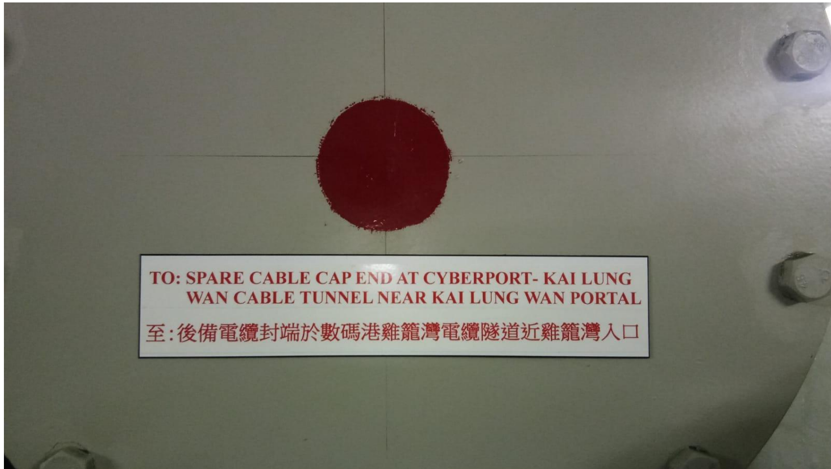
Figure 6. Wordings of New Labels with Additional Information on Cable Connection Tank at CPX
