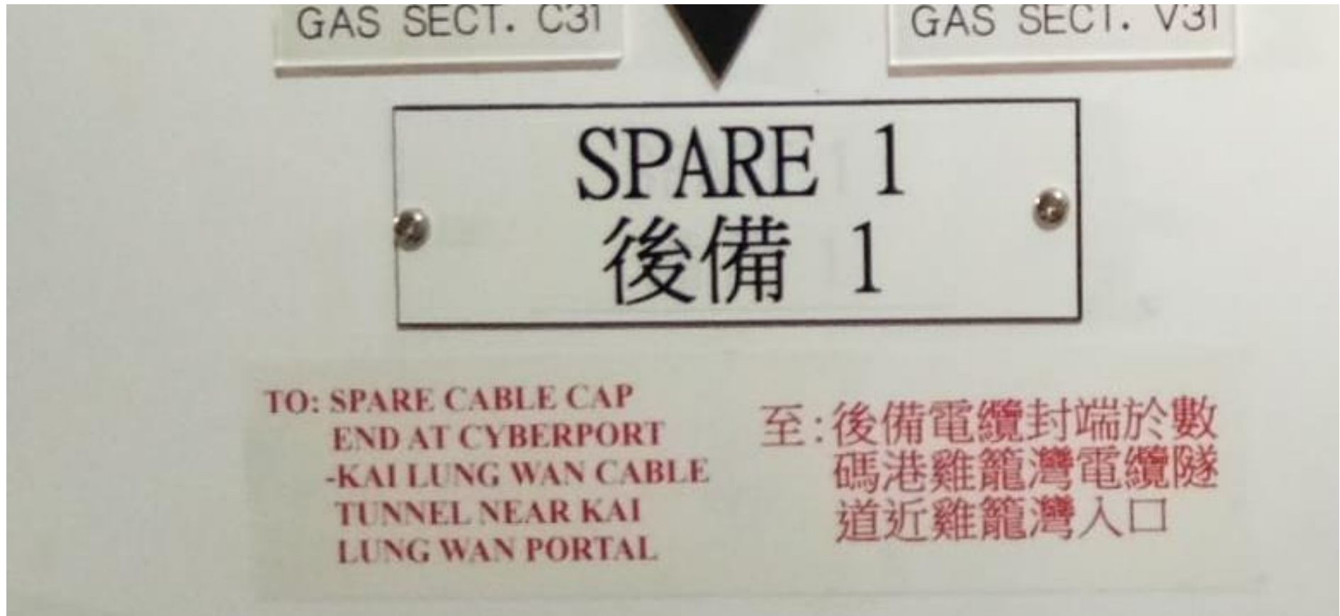
Figure 4. Wordings of New Labels with Additional Information on Local Control Panel at CPX
